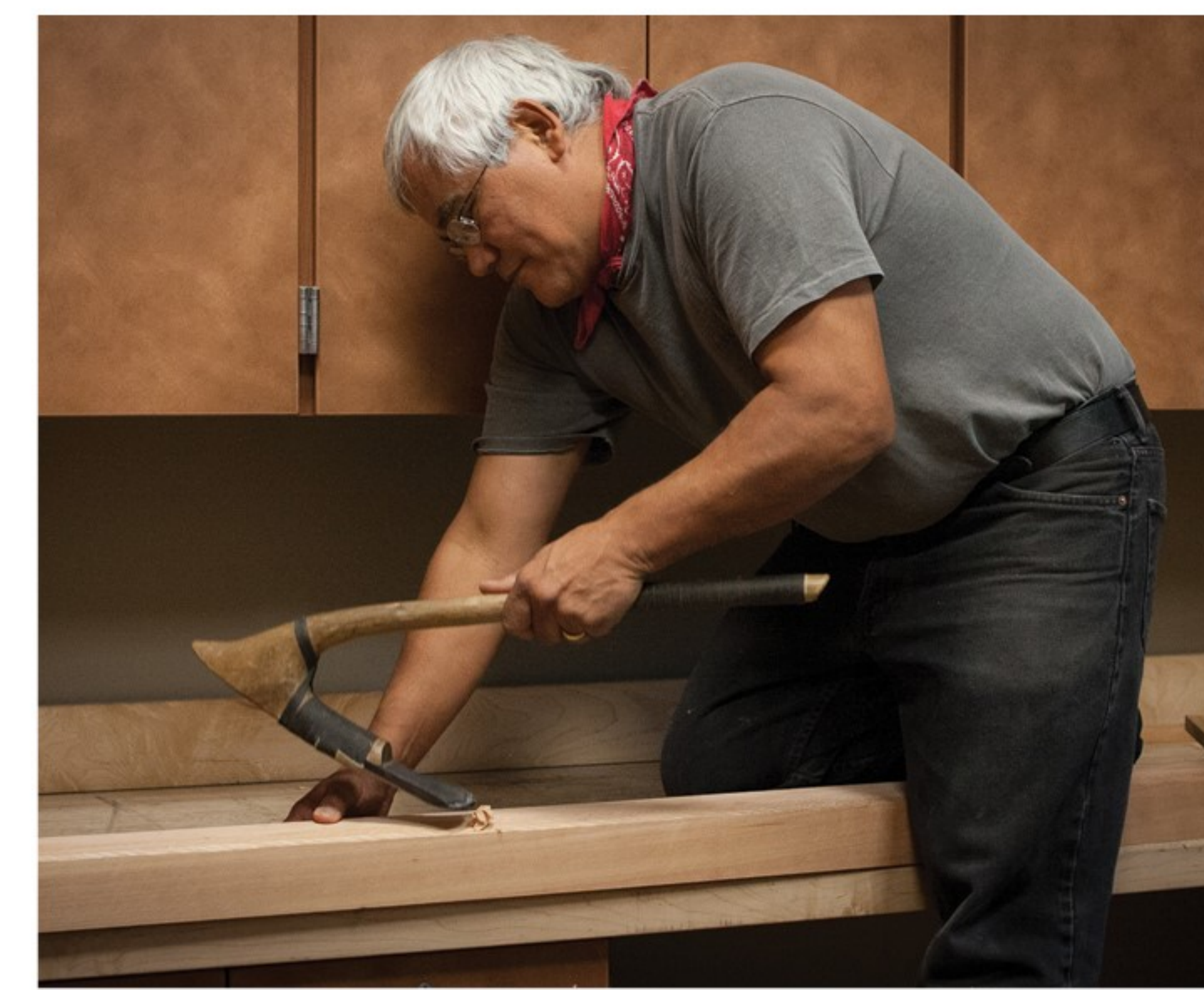
Wayne Price adzing a panel during the construction of the Walter Soboleff Building.
